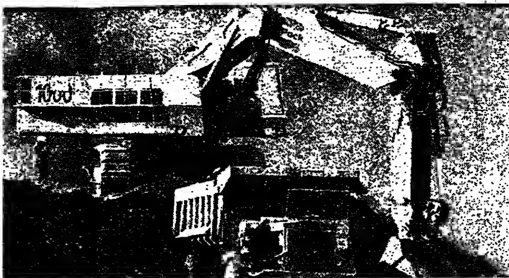
Poclaim 1000CK—the largest hydraulic excavator in the world—working on one of Shand's opencast coalmining sites in South Wales.
